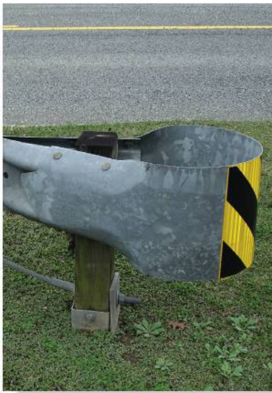
This crash barrier is designed to absorb the impact energy of moving vehicles.
