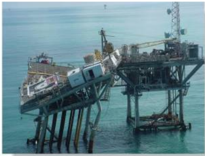
The dramatic failure of this off-shore oil platform was caused by the horizontal forces of hurricane winds, which led to buckling of its supporting columns.
