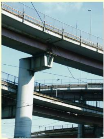
Here is an example of where combined axial and bending stress can occur.
