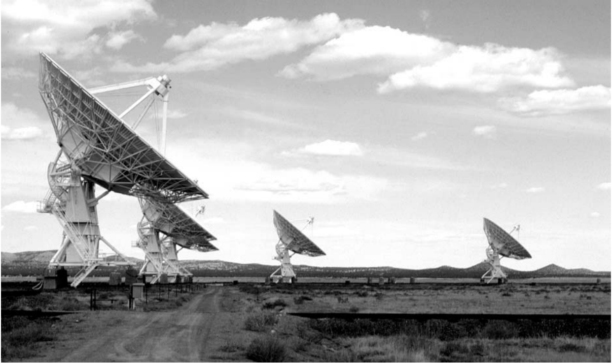
Fig. 3.30. The VLA at Socorro, New Mexico, is a synthesis telescope consisting of 27 movable antennas
